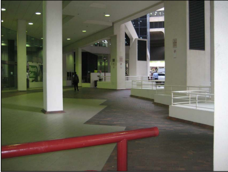
Photograph 1: Facing west and showing the forecourt area of 33-35 Pitt Street. The area is paved.
