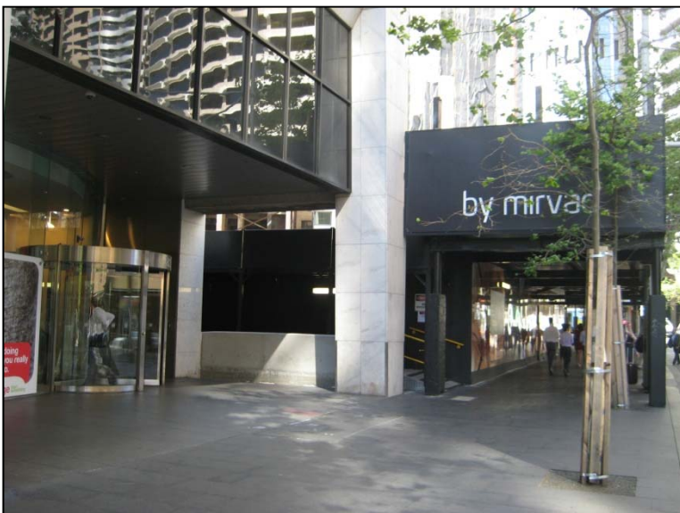
Photograph 7: Facing south east and looking along the front of 182 George Street towards the Mirvac construction site.
